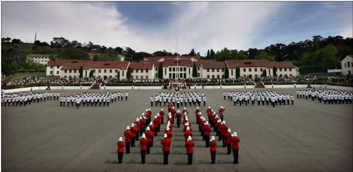
The RMC Duntroon looking north from the main parade ground towards the Sovereign Company barracks, the flag station & the Cadets’ Mess.
